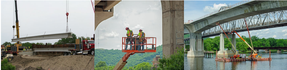
Photos courtesy of MnDOT.
