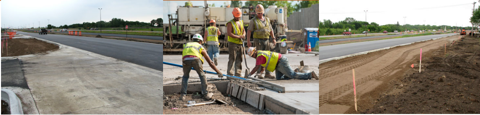
Photos courtesy of MnDOT.
