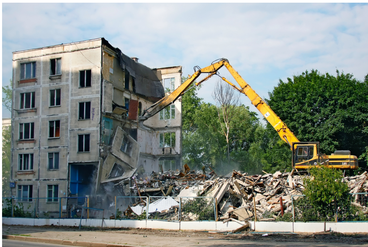
Figure 41: A photo of a building being demolished. In order to align with EO 12898, agencies and jurisdictions receiving Federal funds, including the APO, must take appropriate and necessary steps to identify and address disproportionately high and adverse effects of Federal projects on the health or environment of people-of-color or low-income households to the greatest extent practicable and permitted by law.
