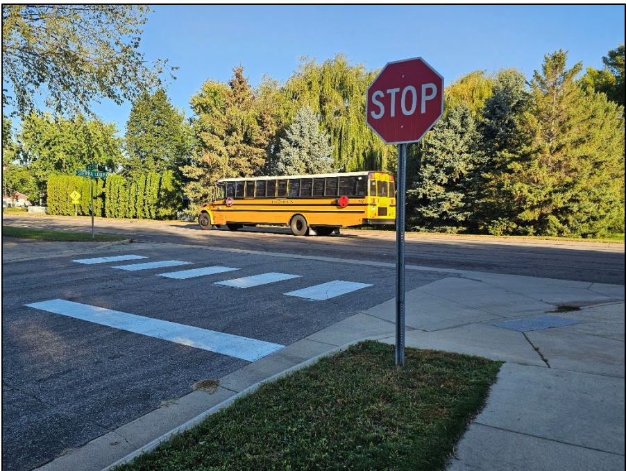
Figure 129. An advanced stop bar at the intersection of 2-1/2 Street N and Sierra Loop.
