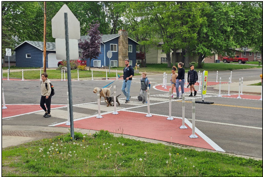
Figure 197. Example of a temporary corner extension in Sauk Rapids.
