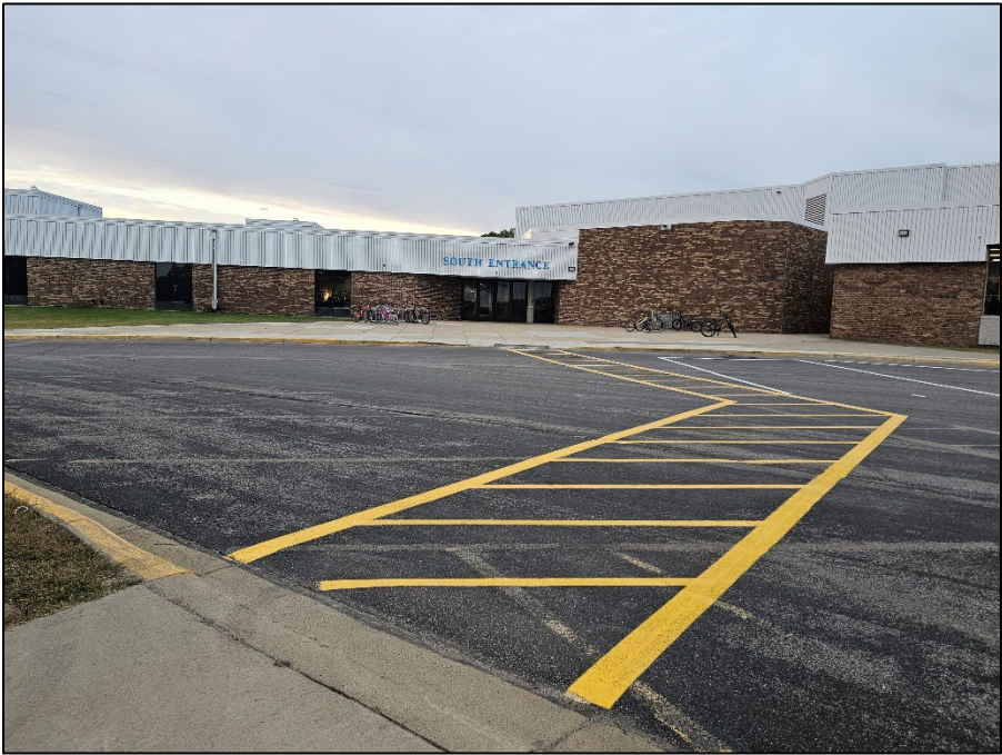
Figure 209. A missing ADA warning surface at a crosswalk at Riverside Intermediate School.
