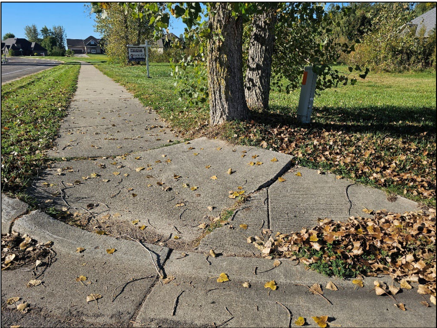
Figure 110. The intersection of 13th Avenue N and Bear Path Court lacks a detectable warning surface.
