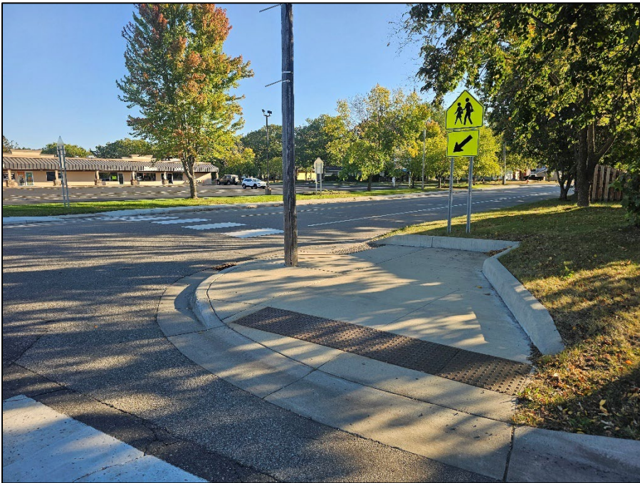
Figure 108. A detectable warning surface at the intersection of Seventh Street N and Second Avenue N.
