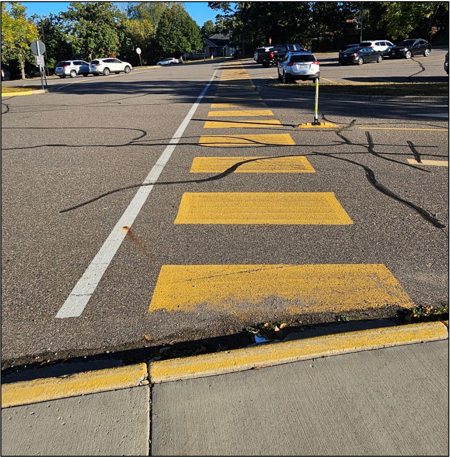
Figure 210. A missing ADA warning surface at a crosswalk at Sartell Middle School.
