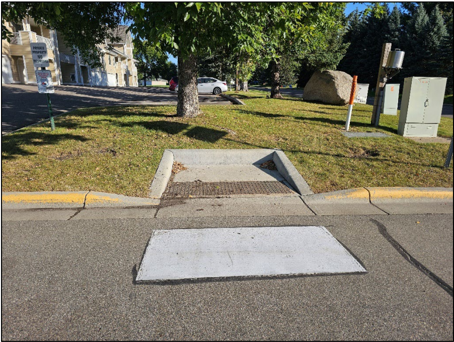
Figure 109. A detectable warning surface at the intersection of Ninth Avenue N and the Sartell Middle School entrance/exit.
