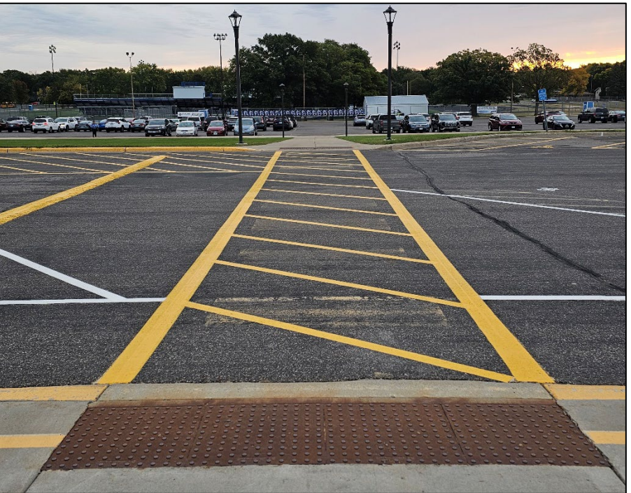
Figure 64. Crosswalk with ADA curb ramp in the Riverview Intermediate School parking lot.
