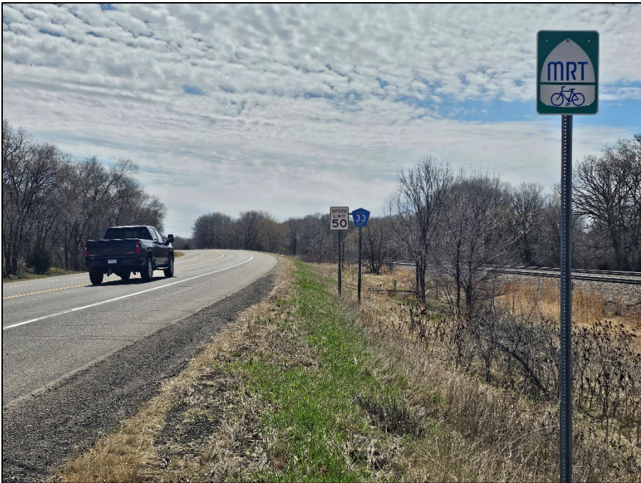
Figure 100. An on-road paved shoulder for bicycles on North Benton Drive.
