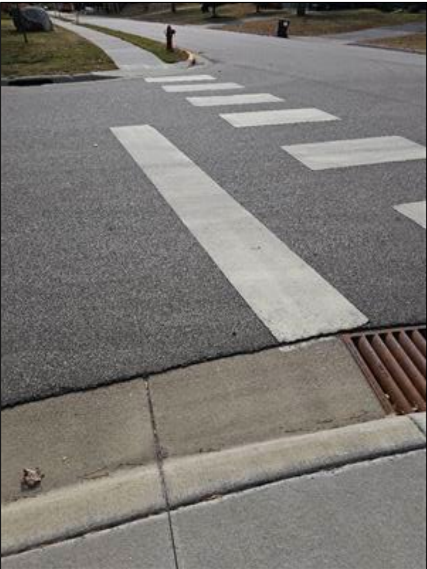
Figure 167. Advanced stop bar at Fifth Street N.
