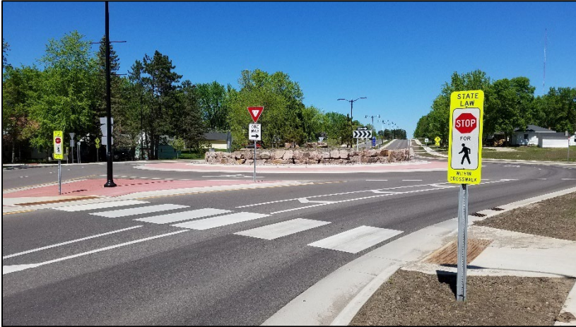
Figure 12: Photo of the roundabout at the intersection of Benton CSAH 3/Second Street N and Sixth Avenue N in Sauk Rapids. Photo courtesy Saint Cloud APO.
