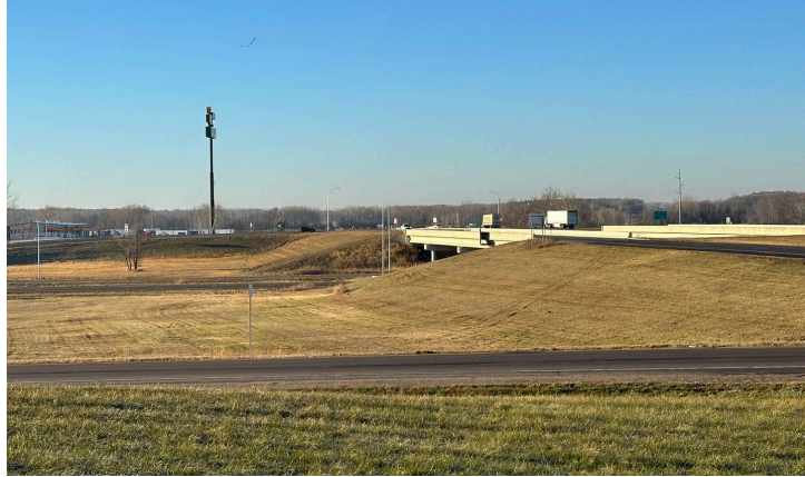
State Highway 23 interchange over I-94, a Principal Arterial Interstate
