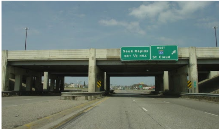
State Highway 10 is an Other Principal Arterial Expressway
