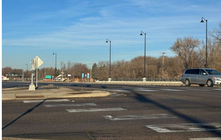
Benton Drive in Sauk Rapids is a Minor Arterial
