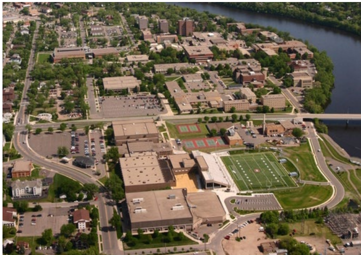
4th Ave. S, adjacent to Saint Cloud State University shown on the left side of this photo is a Major Collector
