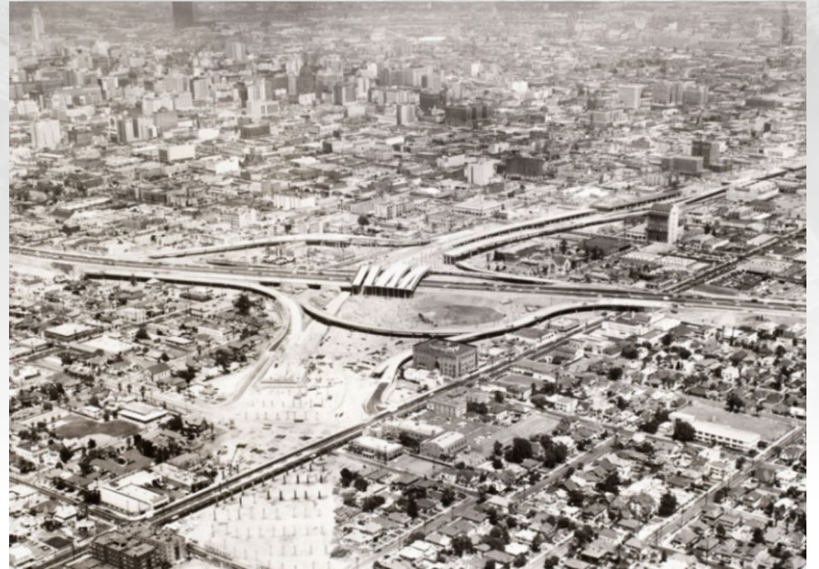
I-10 construction in Los Angeles, 1961
