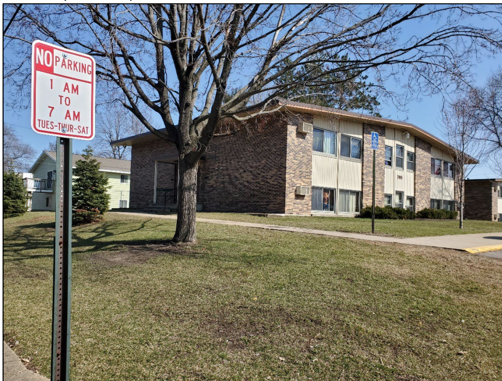
Figure 2.1: Photo of Key Row Community Apartments located in south Saint Cloud. These apartments are located in a Census block group with a large concentration of low-income households. Photo courtesy Saint Cloud APO.
