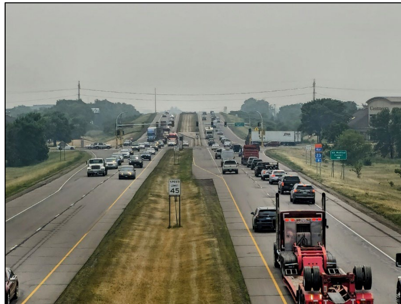
Figure 5.4: MN 15 at the intersection with Veterans Drive/CSAH 4 in Saint Cloud. This roadway, a four-lane divided arterial in an urban/developing area will be at capacity (a V/C ratio of 1.00) if the average annual daily traffic (AADT) exceeds 35,800 vehicles. Current AADT for this section of MN 15 is 32,700 vehicles (a V/C ratio of 0.91). meaning this portion of MN 15 has an LOS E rating. Photo courtesy of Saint Cloud APO.
