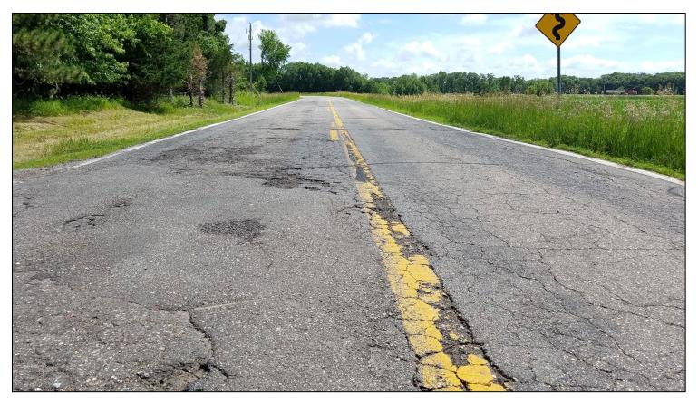
*Figure 4.4:* Cracking pavement along Graniteview Road in Waite Park taken in 2019. Photo courtesy Saint Cloud APO.
