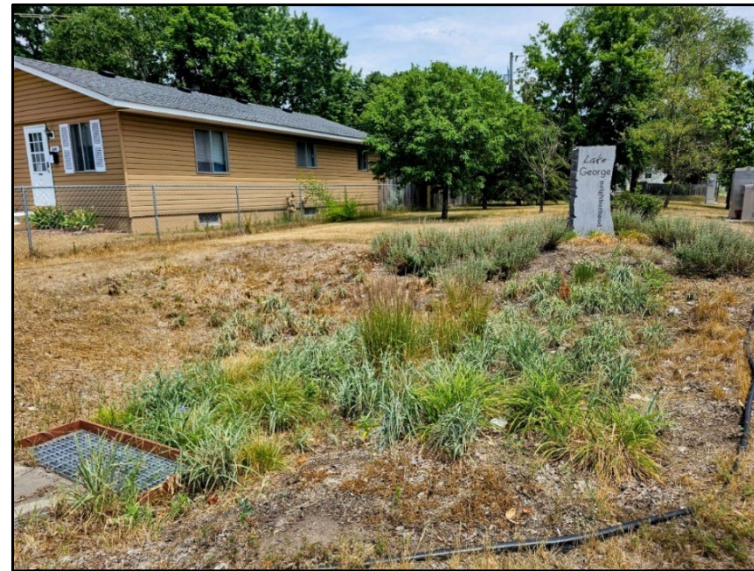
Figure 3.26: Example of a rain garden in the Lake George neighborhood. Photo courtesy of Saint Cloud APO.
