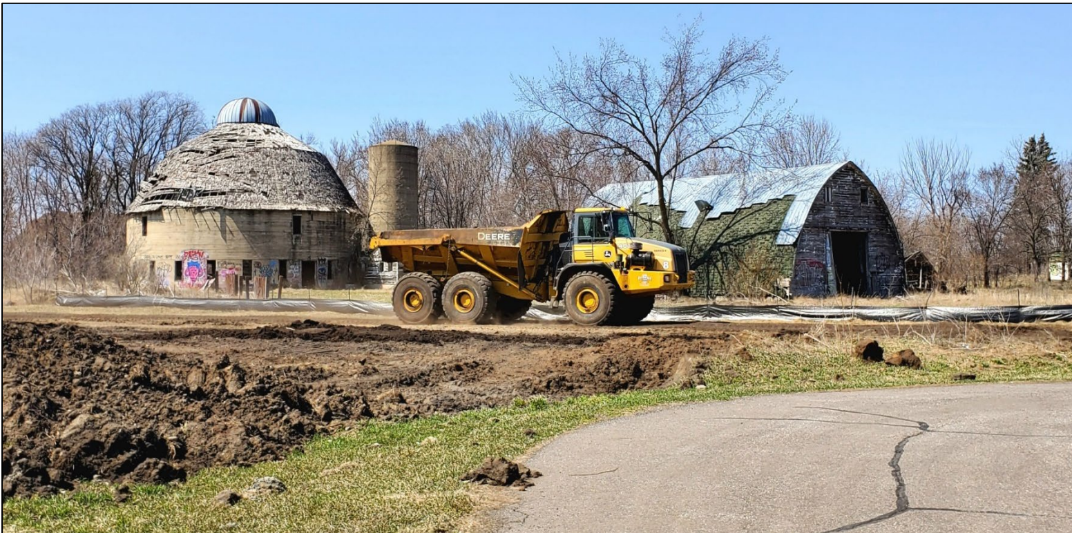
Figure 3.68: Construction of Scout Drive in Sartell. Photo courtesy of Saint Cloud APO.
