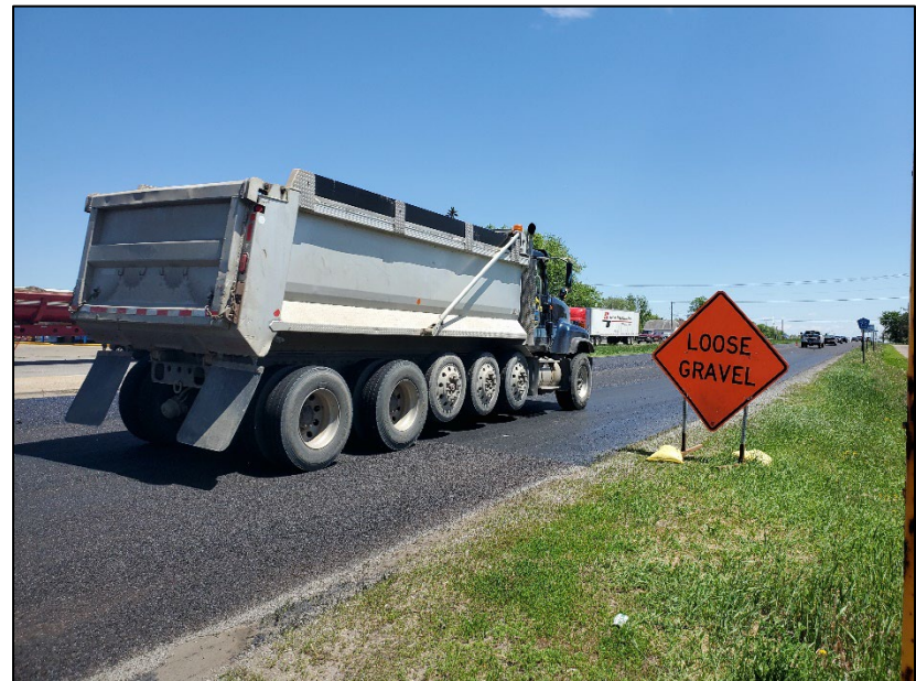
Dump truck traveling along a stretch of Stearns CSAH 75 in Saint Joseph. Photo courtesy of Saint Cloud APO.
