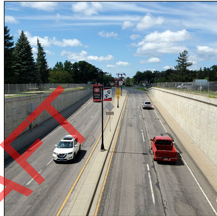
Figure 8.2: A photo of University Drive in Saint Cloud. This roadway is an example of a four-lane, at-grade divided minor arterial. Photo courtesy of Saint Cloud APO.
