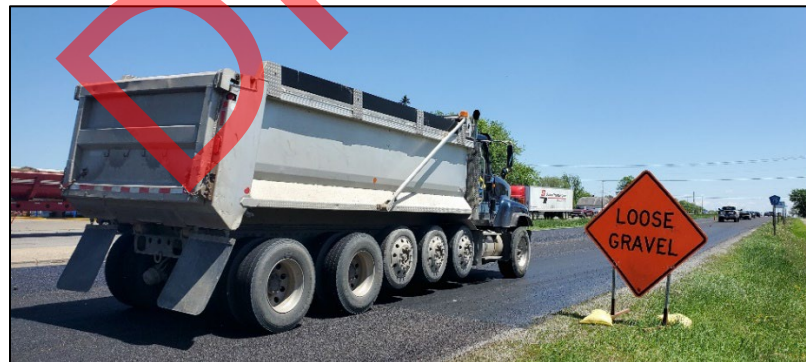
Figure 7.2: Roadway construction along CSAH 75 in Saint Joseph. Photo courtesy of Saint Cloud APO.
