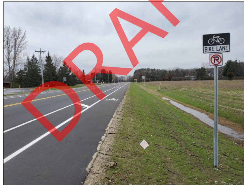
Figure 2.133: Buffered on-road bicycle lane along Oak Grove Road/County Road 136 in Saint Cloud. Photo courtesy Saint Cloud APO.
