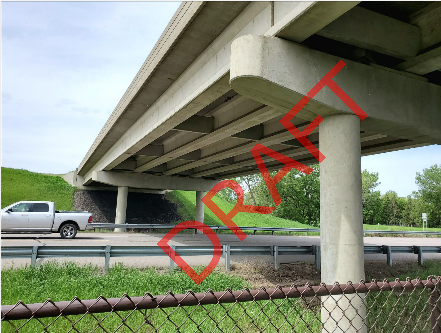
Figure 2.90: I-94 bridge near Saint Joseph. Photo courtesy Saint Cloud APO.
