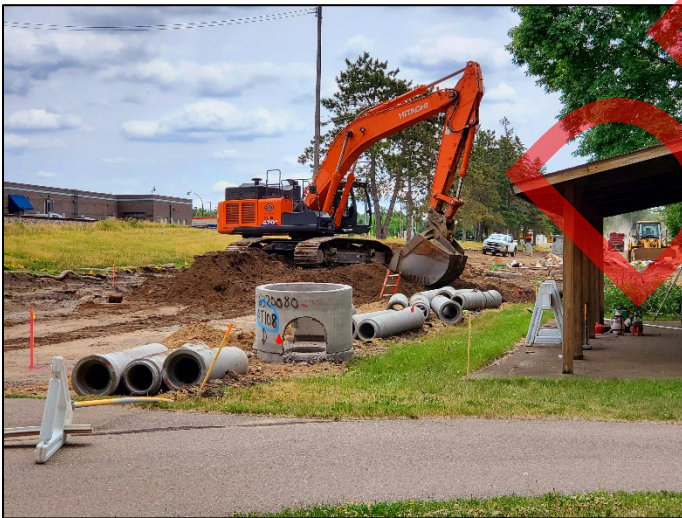
Crews working on reconstructing River Avenue N in Sauk Rapids. Photo courtesy of Saint Cloud APO.
