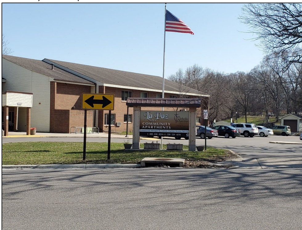
Figure 2.1: Photo of La Pez Community Apartments located in south Saint Cloud – in a Census block group with a large concentration of low-income households. Photo courtesy Saint Cloud APO.
