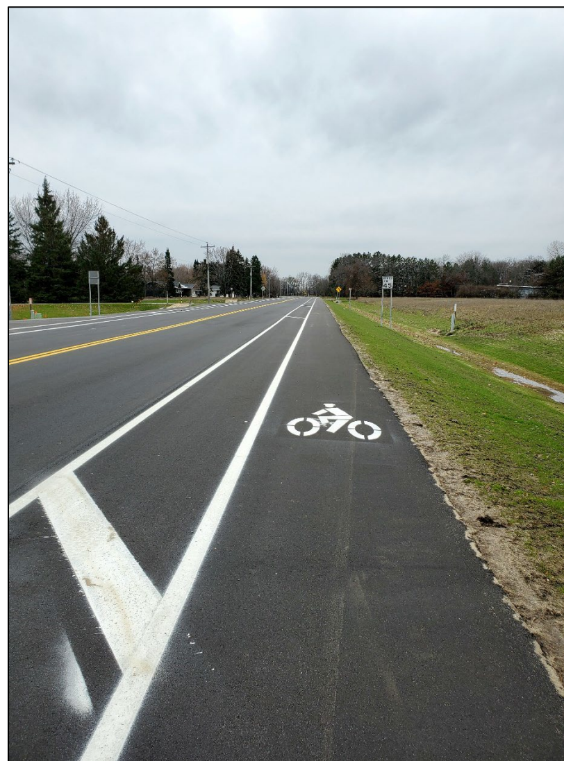
Figure 6.1: Photo of Stearns County Road 136/Oak Grove Road SW. This project, constructed in 2021, received Federal funding to complete.
