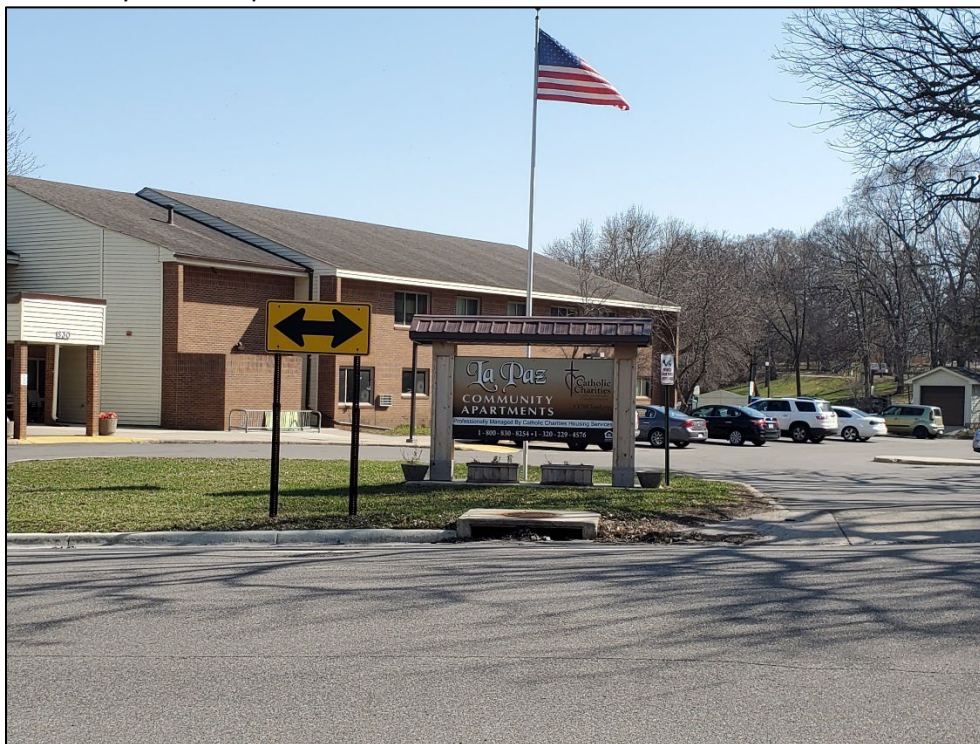
Figure 2.1: Photo of La Pez Community Apartments located in south Saint Cloud – in a Census block group with a large concentration of low-income households. Photo courtesy Saint Cloud APO.
