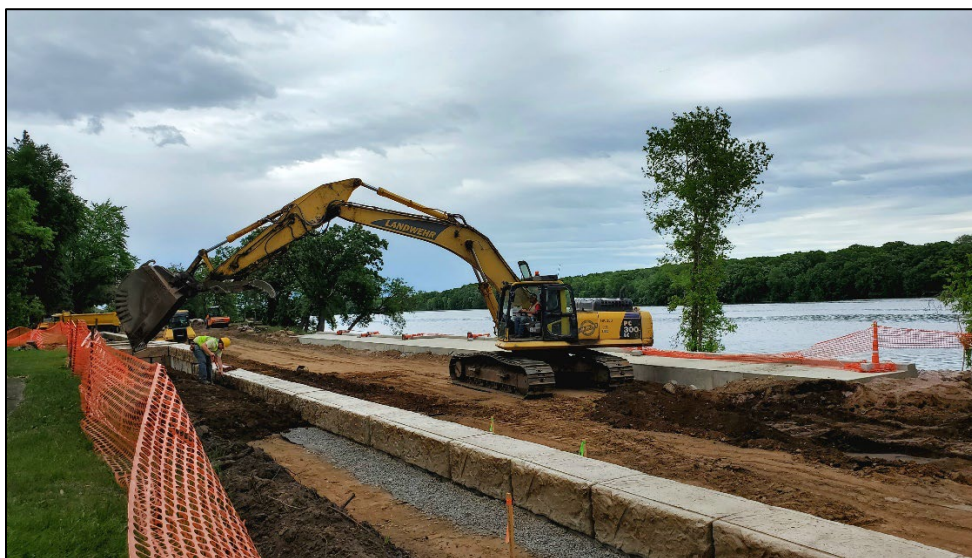
Figure 1.1: An excavator working on the 2022 reconstruction of Stearns County CSAH 1 in Sartell. Photo courtesy Saint Cloud APO.
