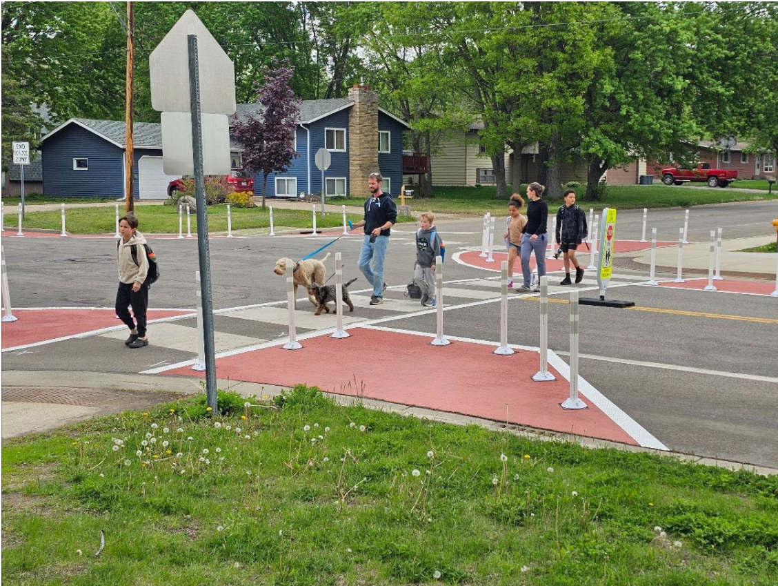
Sauk Rapids residents navigating the temporary curb extensions and pedestrian crossing enhancements at the intersection of 11th Street N and Sixth Avenue N in Sauk Rapids. Photo courtesy of Saint Cloud APO.
