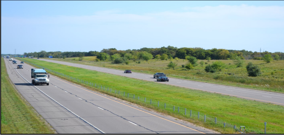
Interstate 94 in Saint Cloud. Photo courtesy of the APO.
