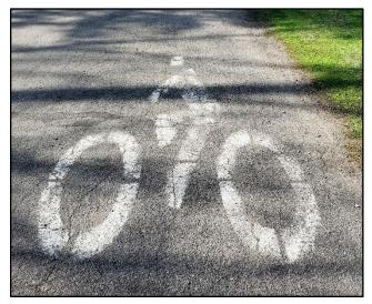
Figure 60. Example of a shared lane bike marking.
