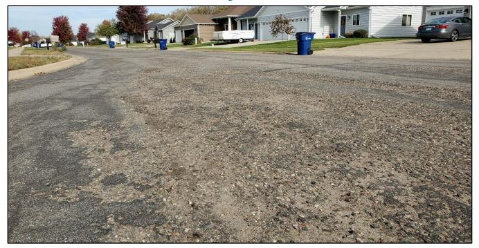
Figure 44. Example of poor pavement condition on Glad View Court.
