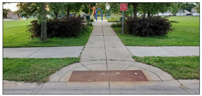
*Figure 38. Example of a detectable warning surface on a curb ramp.*
