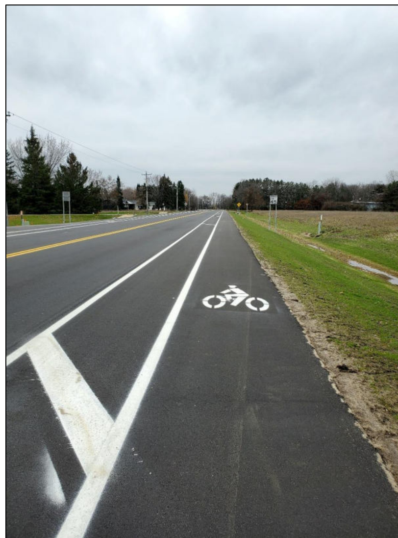
Figure 6.1: Photo of Stearns County Road 136/Oak Grove Road SW. This project, constructed in 2021, received Federal funding to complete.
