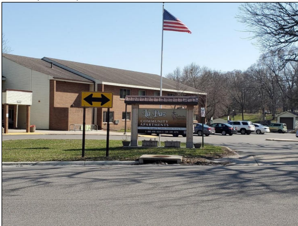
Figure 2.1: Photo of La Paz Community Apartments located in south Saint Cloud – in a Census block group with a large concentration of low-income households. Photo courtesy Saint Cloud APO.
