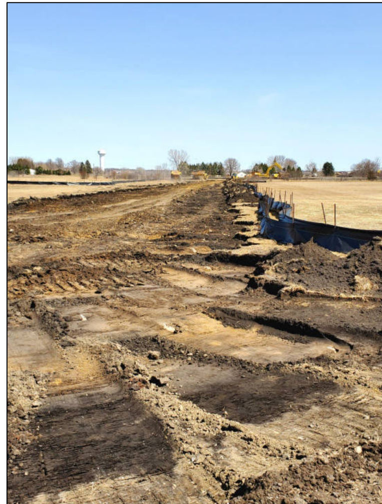
Figure I.5: Scout Drive to Connecticut Avenue S expansionary project construction. Photo courtesy Saint Cloud APO.
