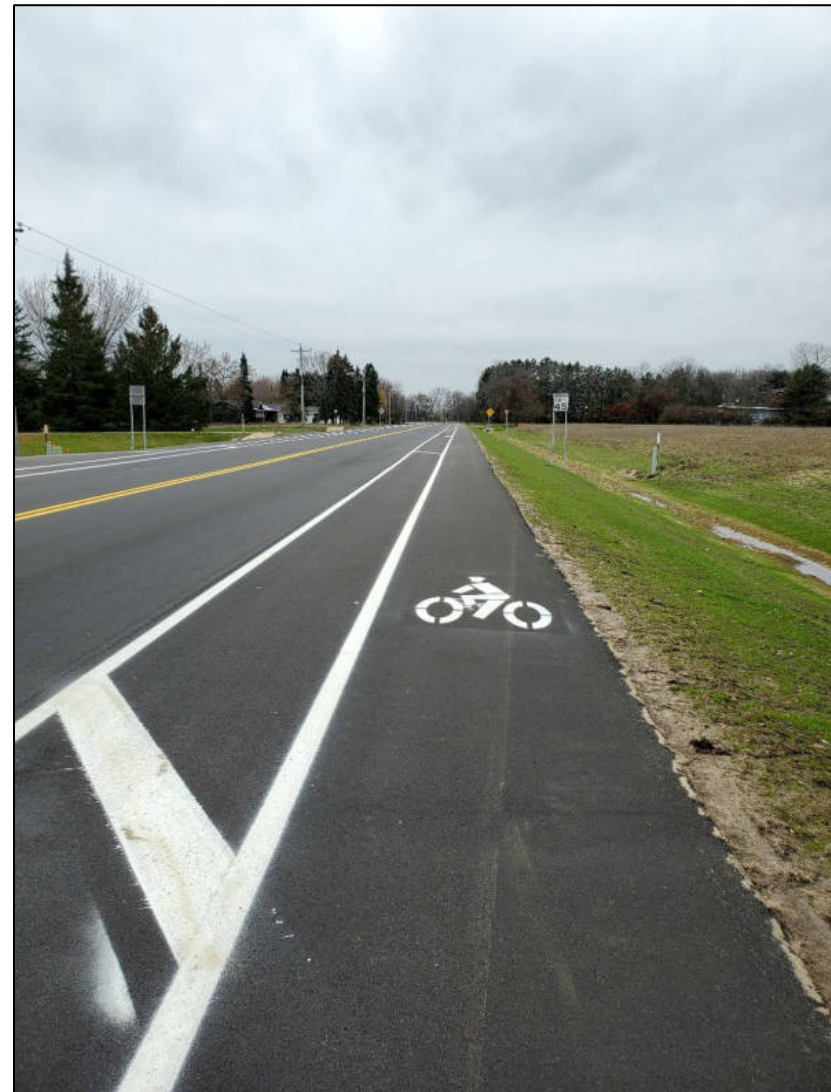
Figure 6.1: Photo of Stearns County Road 136/Oak Grove Road SW. This project, constructed in 2021, received Federal funding to complete.
