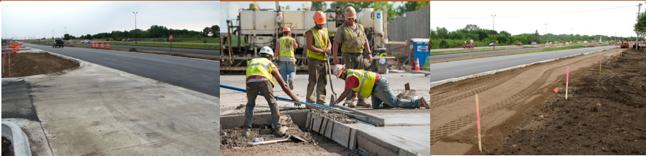
Photos courtesy of MnDOT.
