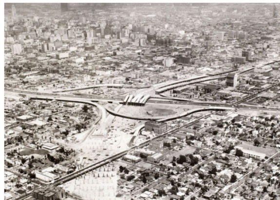
I-10 construction in Los Angeles, 1961
