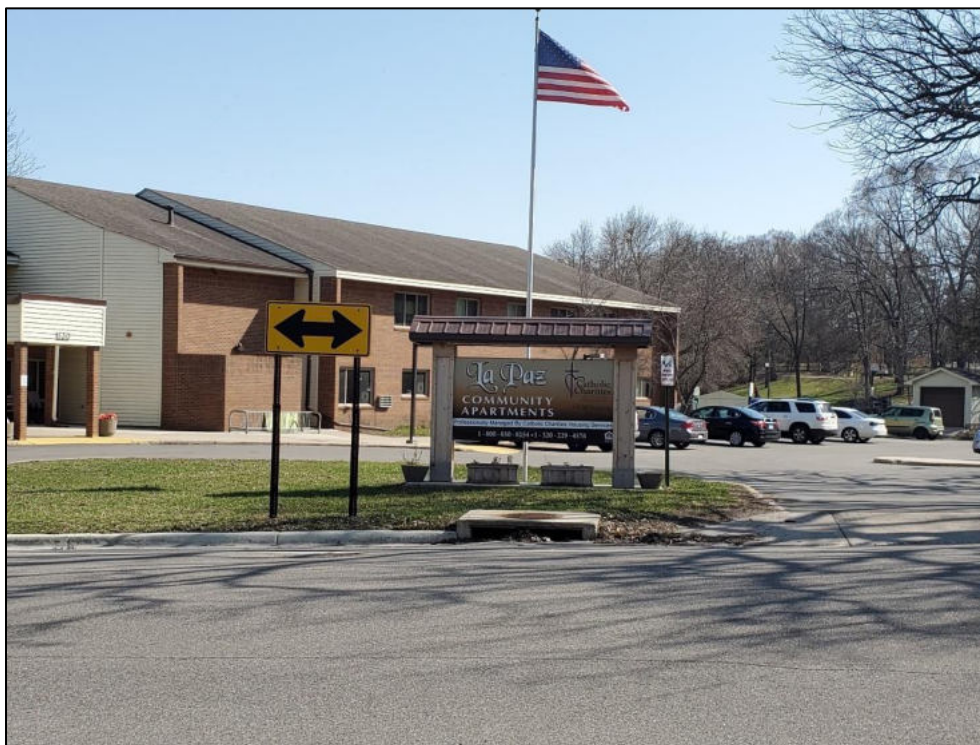
Figure 2.1: Photo of La Pez Community Apartments located in south Saint Cloud – in a Census block group with a large concentration of low-income households. Photo courtesy Saint Cloud APO.
