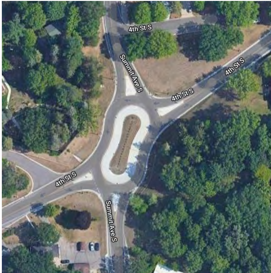
Image ES 2 – Example Bowtie Roundabout (Existing Bowtie Roundabout in City of Sauk Rapids)
