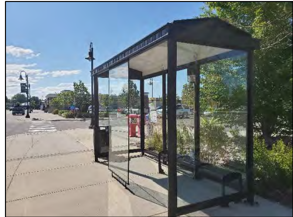
FIGURE 2.12 – A SHELTER AT A TRANSIT STOP.
