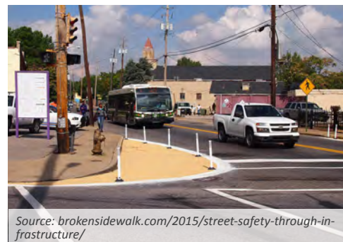
ABOVE Temporary bumpout: mill and overlay
