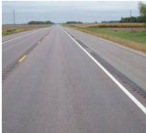
Source: MnDOT. http://www.dot.state.mn.us/trafficeng/safety/rumble/images/RumbleBars.jpg
