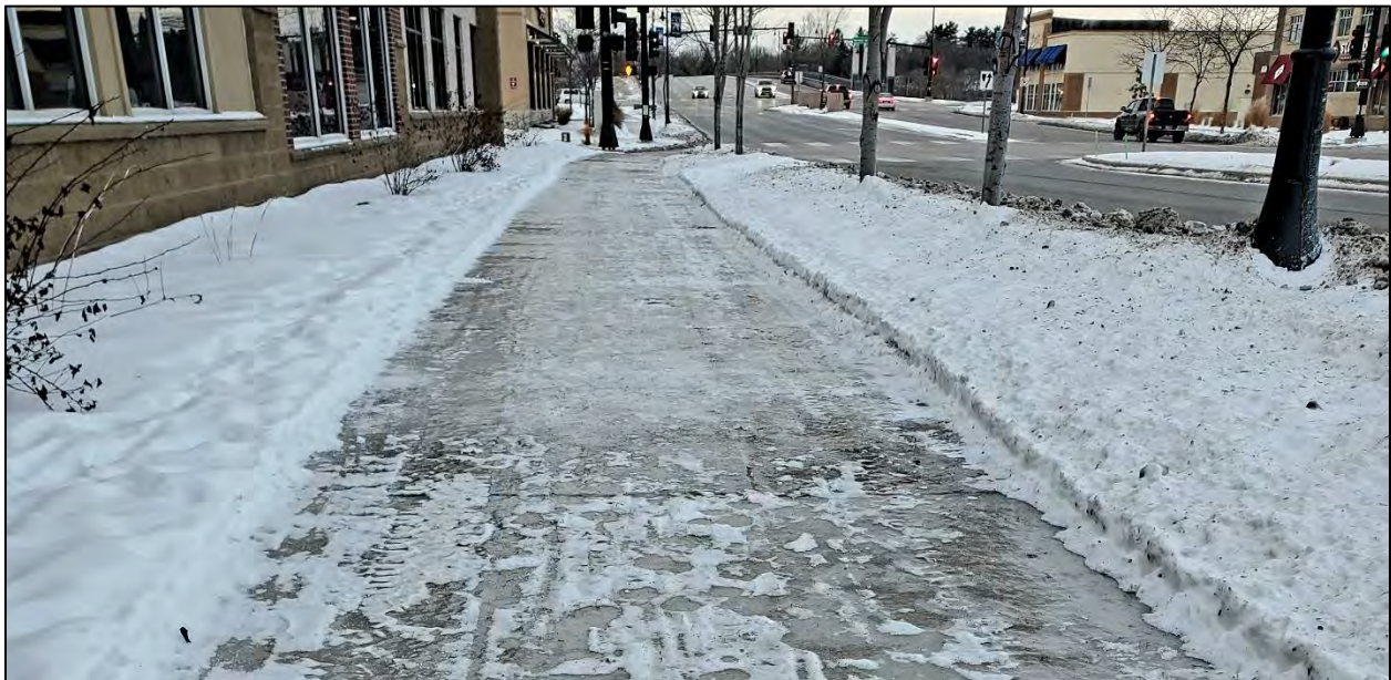
FIGURE 5.5 – EXAMPLE OF AN ICY SIDEWALK IN SAUK RAPIDS.
