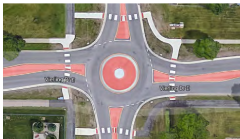
Mini-roundabout in Shakopee, MN. Source: https://www.google.com/maps/@44.7834643,-93.5201076,115m/data=!3m1!1e3
