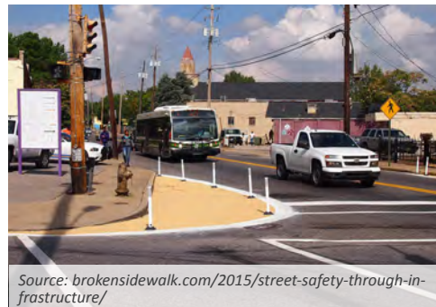
ABOVE Temporary bumpout: mill and overlay
