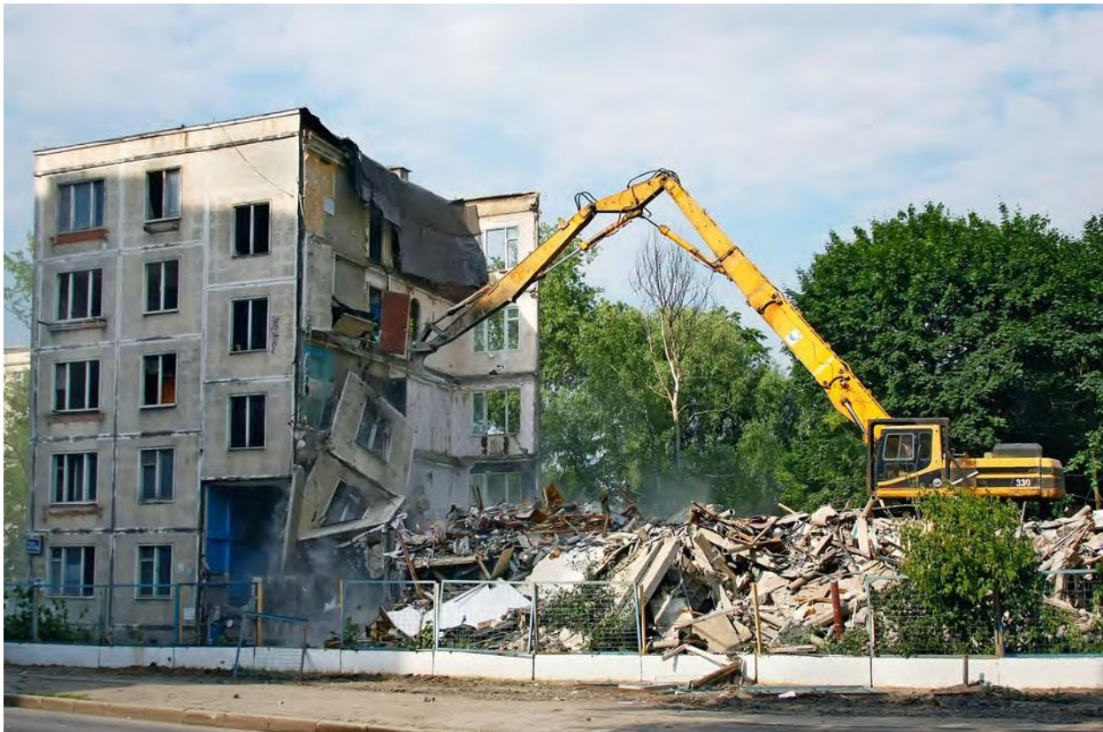
Figure 42: A photo of a building being demolished. In order to align with EO 12898, agencies and jurisdictions receiving Federal funds, including the APO, must take appropriate and necessary steps to identify and address disproportionately high and adverse effects of Federal projects on the health or environment of BIPOC or low-income households to the greatest extent practicable and permitted by law.
