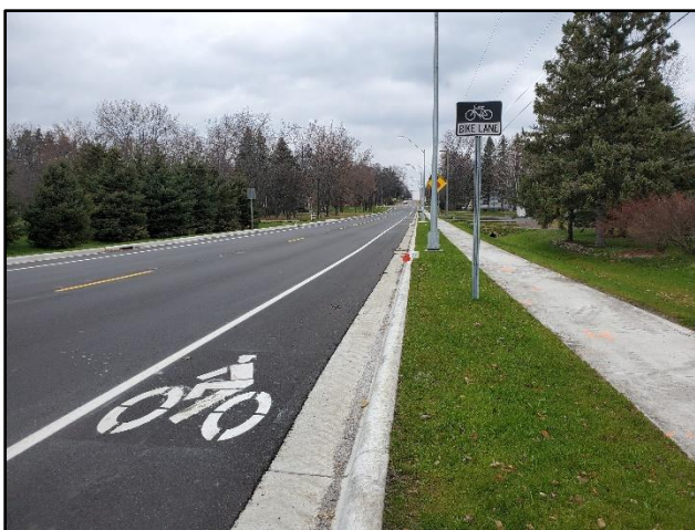
Figure 21. Example of bike lane and sidewalk on Oak Grove Road.
