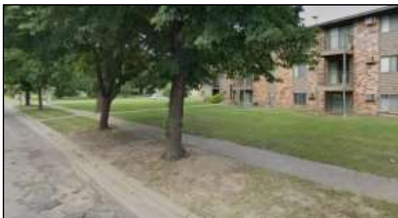
FIGURE 2.7 – AN EXAMPLE OF A SIDEWALK.
