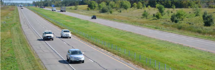
Interstate 94 in Saint Cloud. Photo courtesy of the APO.
