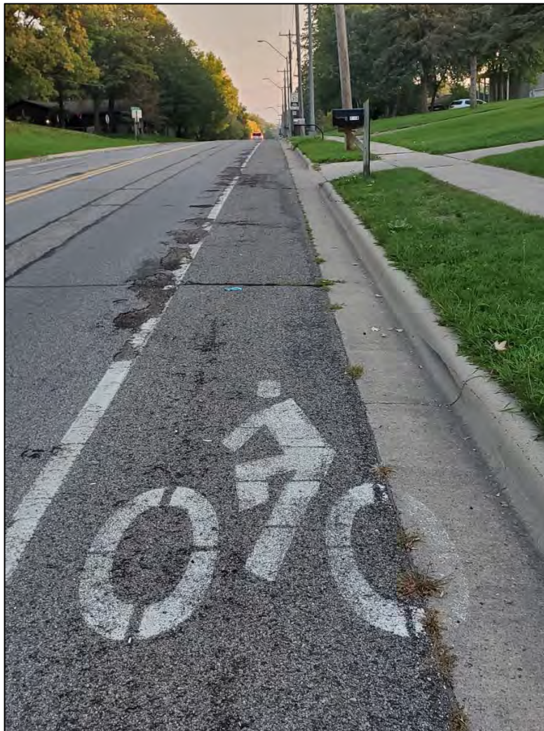
FIGURE E.6 – BIKE LANE ON OAK GROVE ROAD IN SAINT CLOUD.
