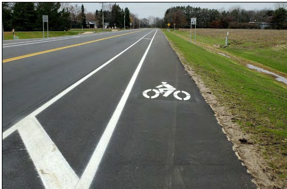
FIGURE E.20 – BUFFERED BIKE LANE ON OAK GROVE ROAD IN SAINT CLOUD.
