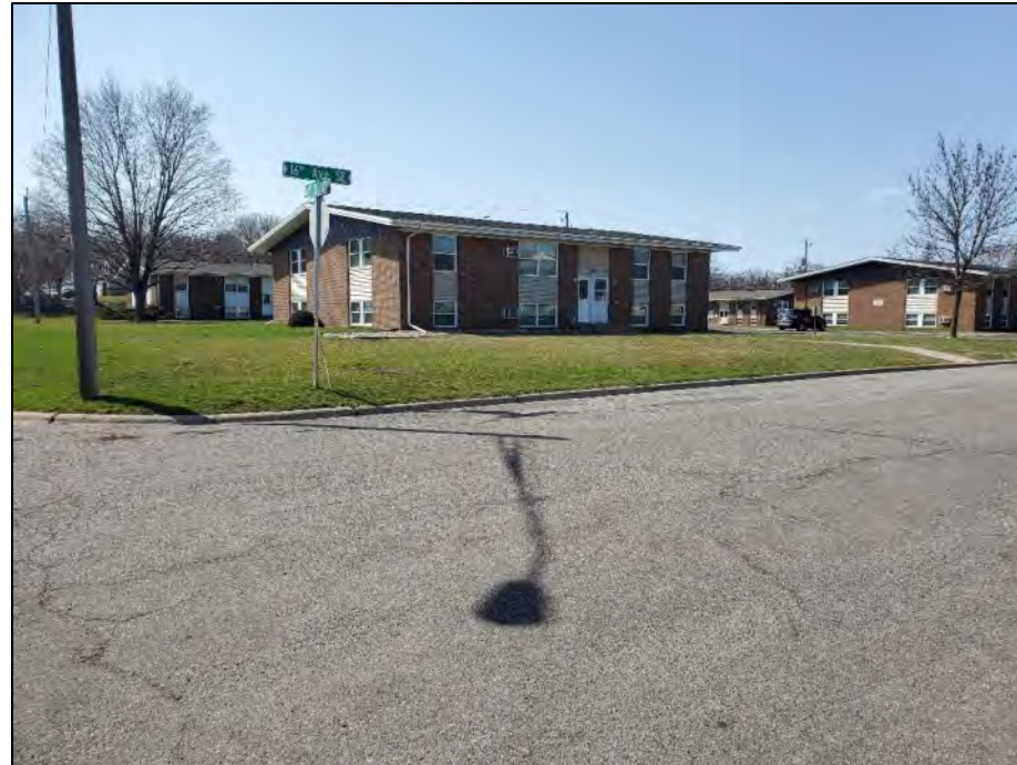
Figure 2.10: A photo of apartment buildings located in southeast Saint Cloud in an area with a higher percentage of low-income and BIPOC populations.
