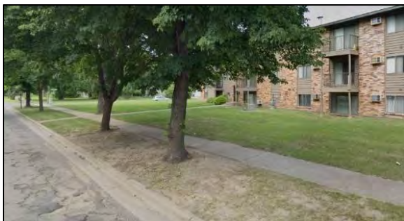
FIGURE 2.7 – AN EXAMPLE OF A SIDEWALK.
