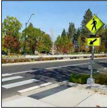
FIGURE 2.5 – AN EXAMPLE OF AN RRFB. PHOTO COURTESY OF AZDOT.GOV.
