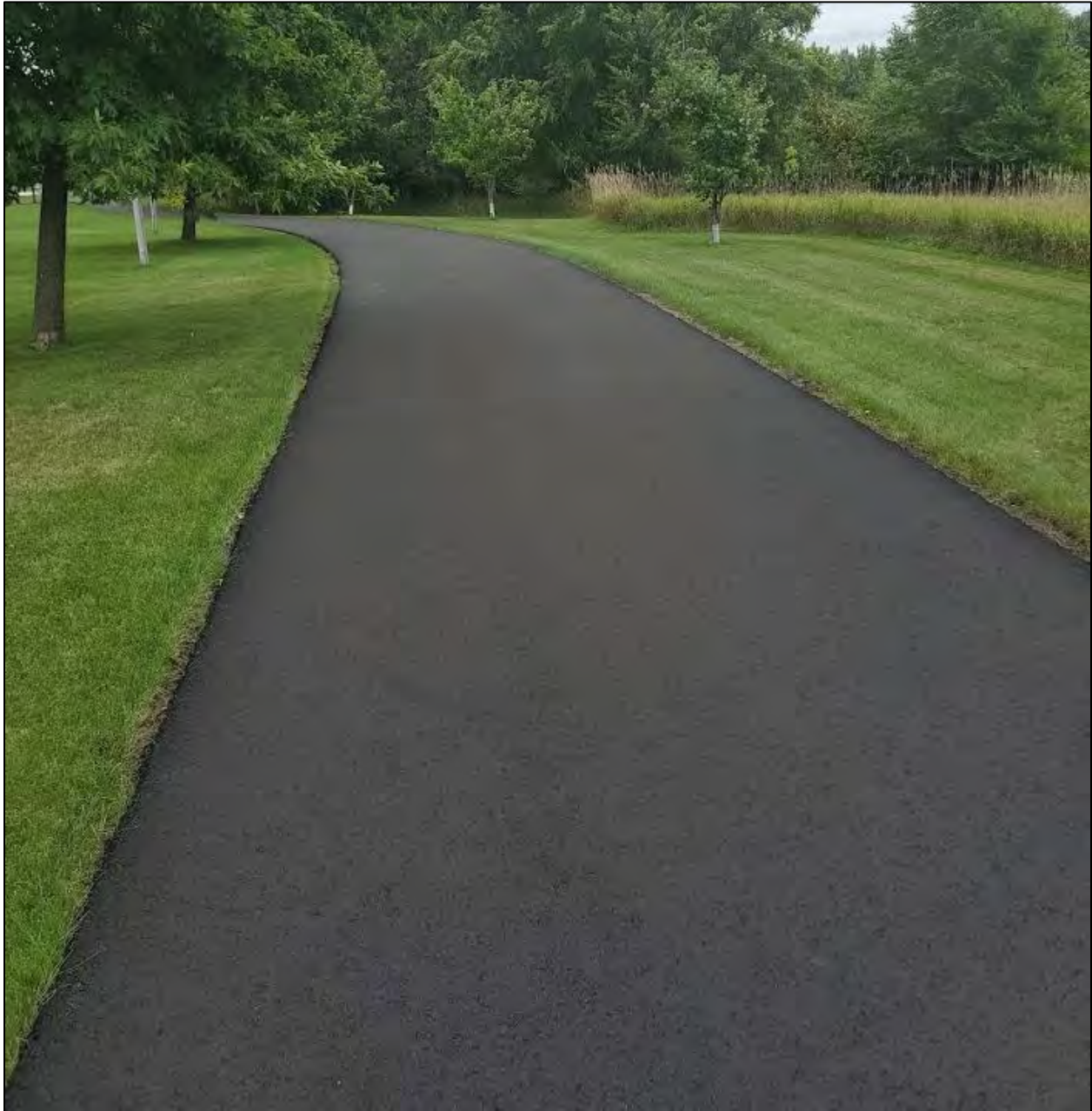
FIGURE 5.4 – EXAMPLE OF A NEWLY PAVED SHARED USE PATH IN SAINT CLOUD
