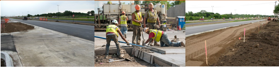
Photos courtesy of MnDOT.
