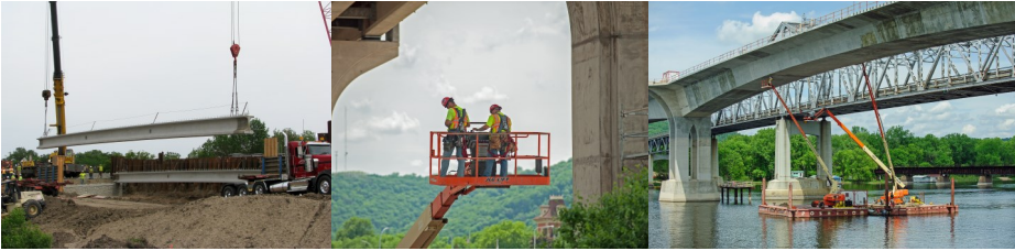
Photos courtesy of MnDOT.
