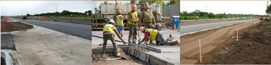
Photos courtesy of MnDOT.
