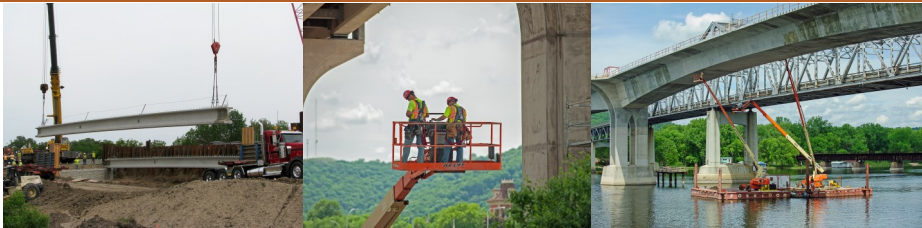
Photos courtesy of MnDOT.
