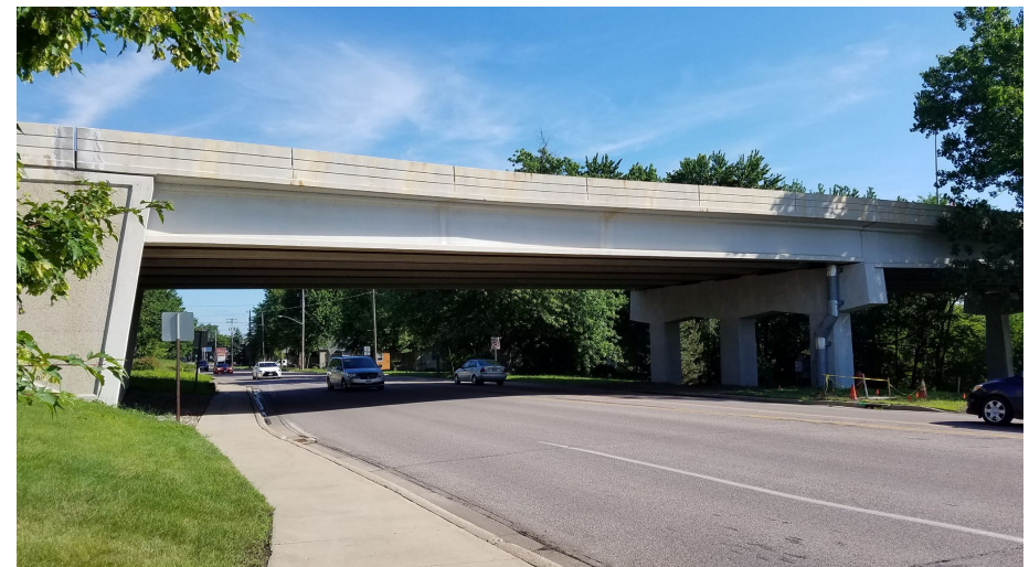
Sartell bridge rated in fair condition. Photo courtesy of the APO.
