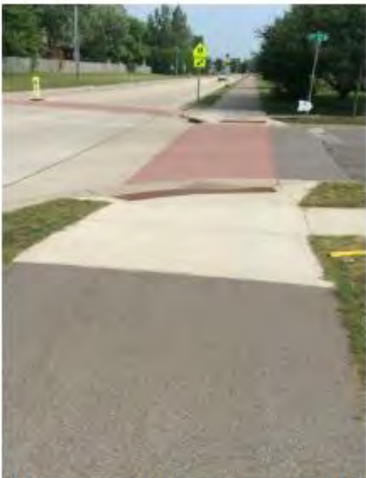
Photo 8 4 th Street N/Pine Cone Road –Fan Ramp, Replacement Urgency 3, Landing Slope
