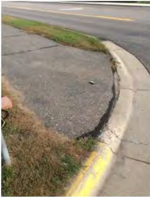
Photo 1 Sartell Lane/2 nd Street South – One Way Directional Ramp, Replacement Urgency 1, No Domes, Slope, Vertical Compliance
