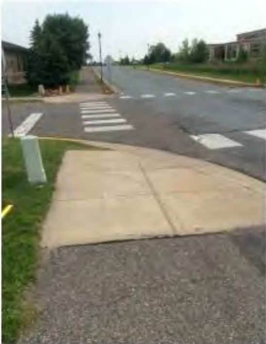
Photo 4 19 th Street S/Connecticut Avenue – Fan Ramp, Replacement Urgency 2, Domes, Slope, Vertical Compliance
