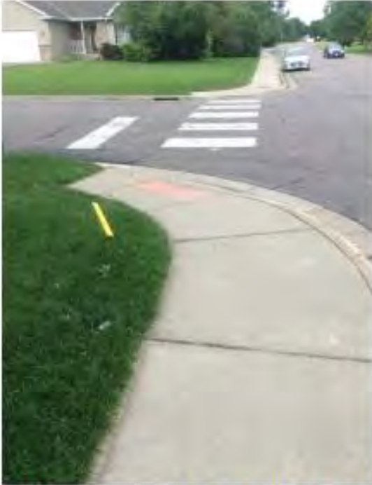
Photo 5 15 th Street N/5 th Avenue N – One Way Directional Ramp, Replacement Urgency 2, Dome width, Slope, Landing
