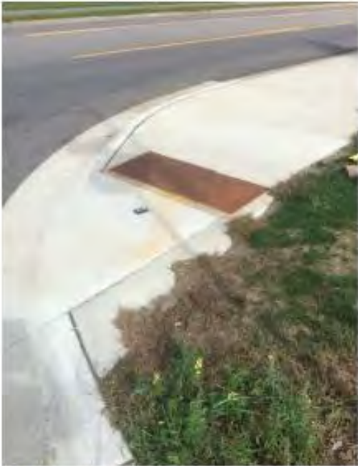
Photo 7 2 nd Street S/Sundance Road – One Way Directional Ramp, Replacement Urgency 3, Dome Width
