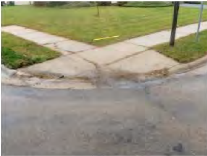
Photo 2 10 th Avenue N/4 th Street N – Fan Ramp, Replacement Urgency 1, No Domes, Landing, Slope, Vertical Compliance
