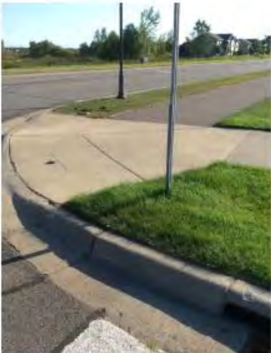
Photo 6 15 th Street S/Lavendar Avenue S – Fan Ramp, Replacement Urgency 2, Domes, Vertical Compliance
