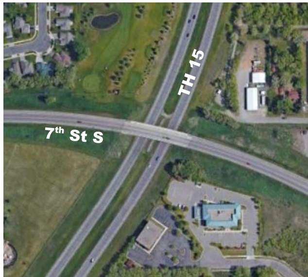
Figure 65 - Buildings Near TH 15 and 7 th Street South
