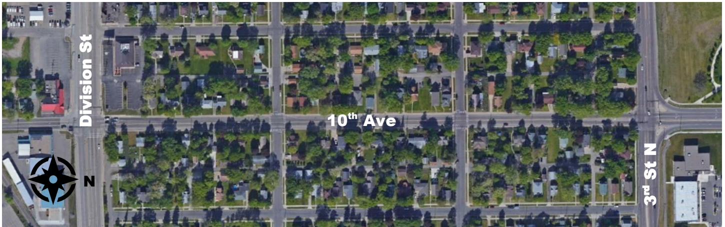
Figure 63 - Potential Access Challenges on 10 th Avenue
