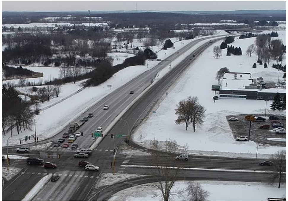
Figure 16 - TH 15 and 2nd Street Intersection Is First Signalized Intersection
