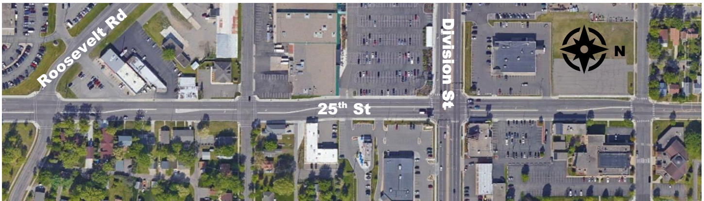
Figure 62 - Potential Access Challenges on 25th Street
