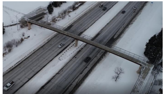
Figure 7 - Pedestrian Bridge connecting Apollo High School
