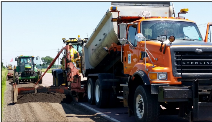
Photo courtesy of MnDOT
